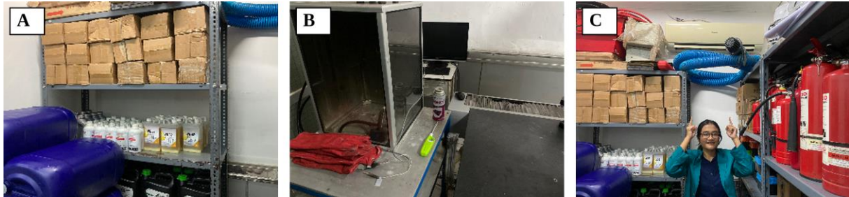
Figure 2. Storage-related hazards: (A) chemicals stored without adequate segregation; (B) flammable gas located near an ignition source; (C) items placed on high racks without adequate restraint.
