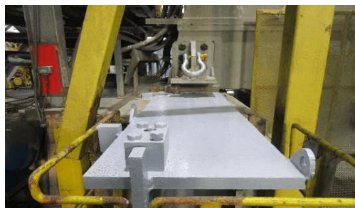
Figure 5. The top coat application
