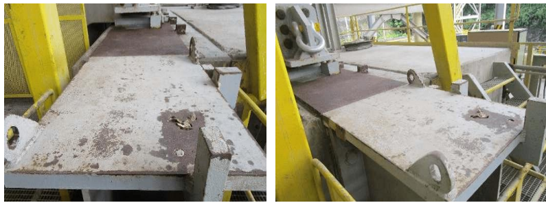
Figure 1. Condition of the plant to be coated
