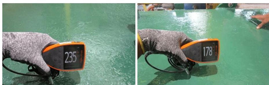
Figure 4. The primer coat application
