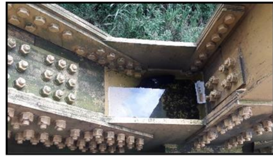
Figure 6. Puddle in joint BB18 left and GD18 left
