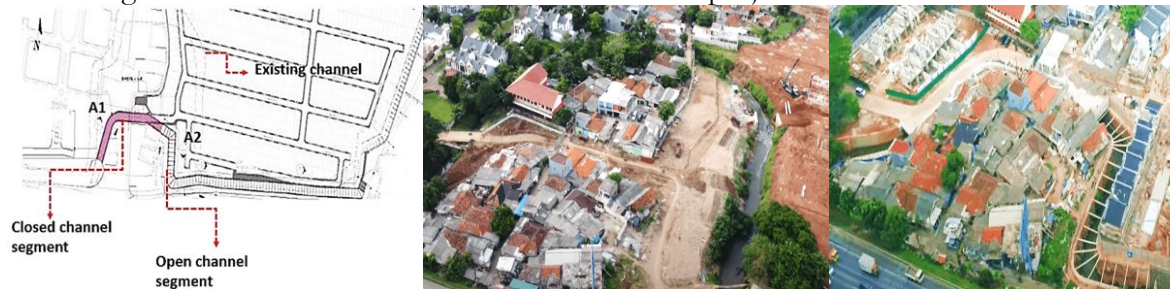
Figure 1. Overview of the channel diversion
