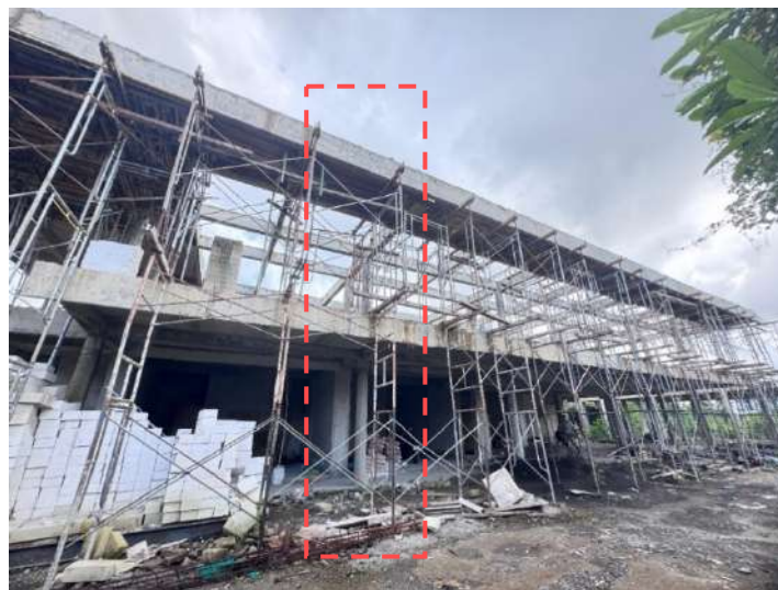
Figure 1. Existing Structure of the Cantilever Beam without Strengthening
