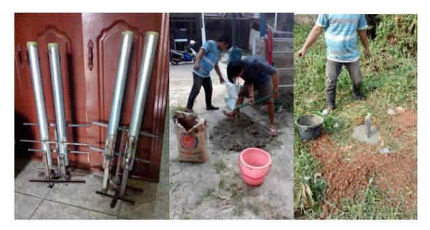
**Figure 5.** Installation of Foundations for PV Mini-Grid Light Poles
