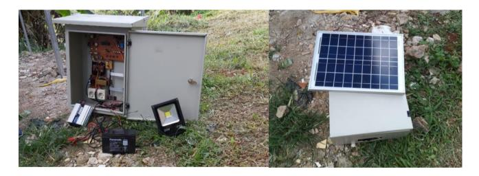
**Figure 3.** Components and Parts of PV Mini-Grid
