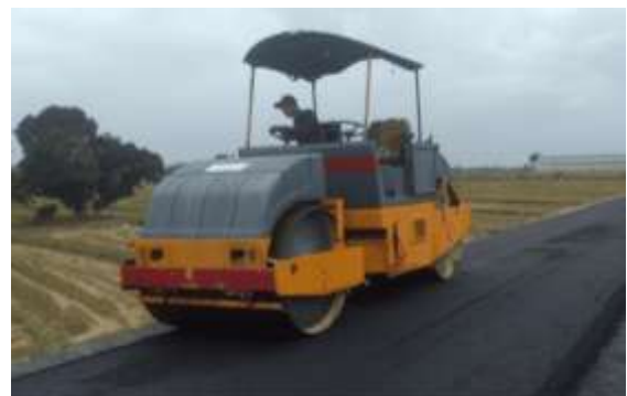
Gambar 11. Pekerjaan Surface Course
