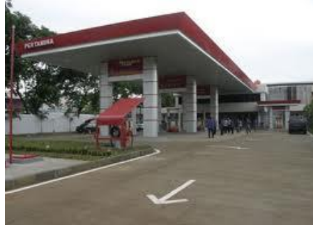
Gambar 6. SPBU RTH Kapuk
