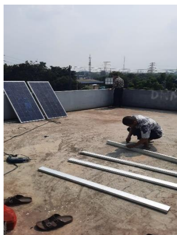
Gambar 6. Proses perakitan Solar Panel
